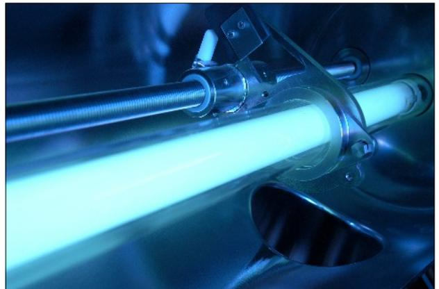
Ozone gas is also sucked through the exhaust ducts breaking down any grease that has collected deeper inside the ductwork. Another benefit is that the Ozonolysis process has the effect of deodorizing the exhaust air- an increasing requirement in many countries.
